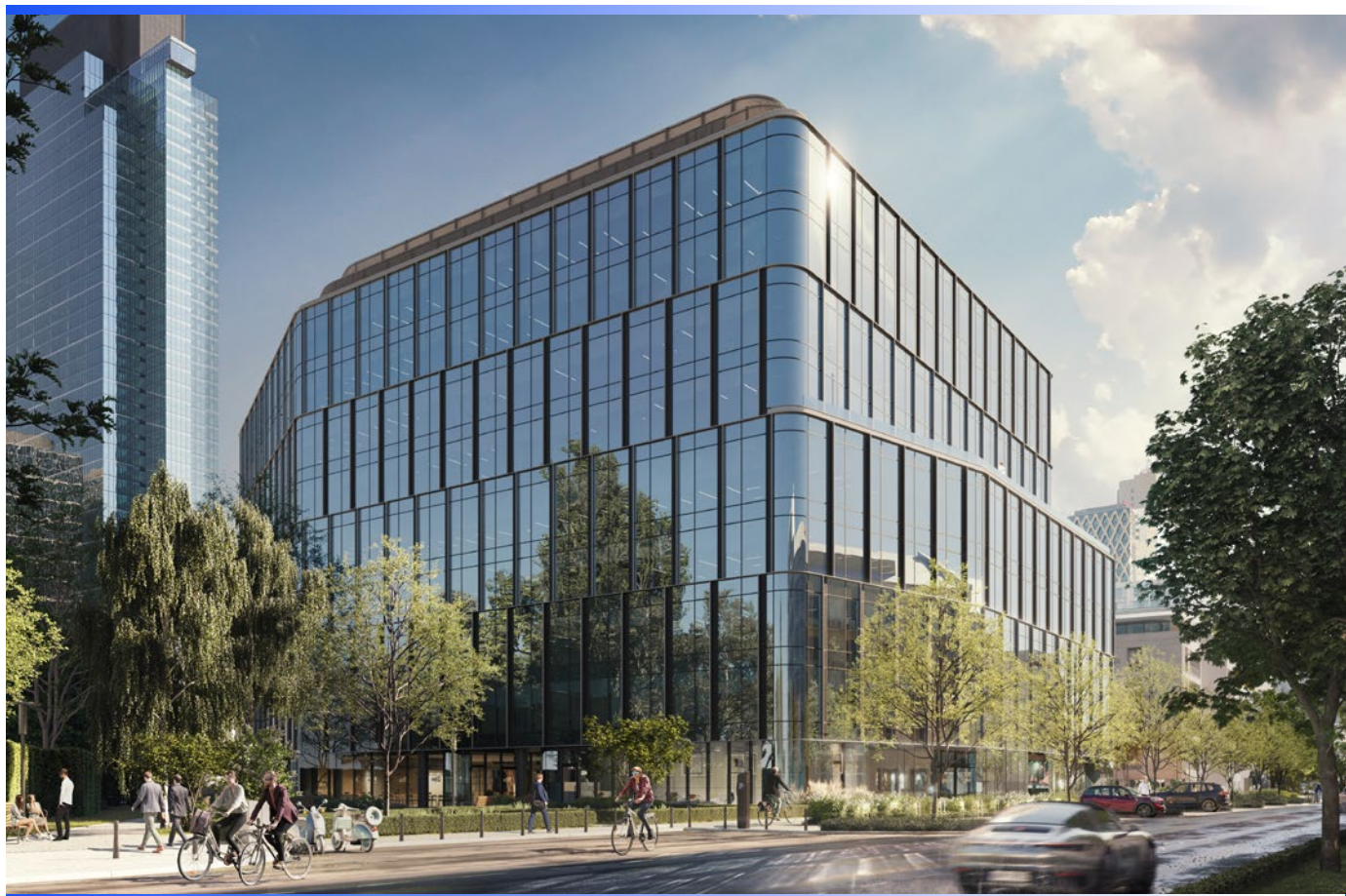
Budynek The FORM, Warszawa, Lincoln Property Company
